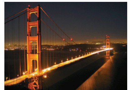
s / The Golden Gate Bridge's roadway is held up by the tension in the vertical cables.
